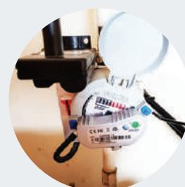
FIG. 6: AMR-enabled inductive meter
