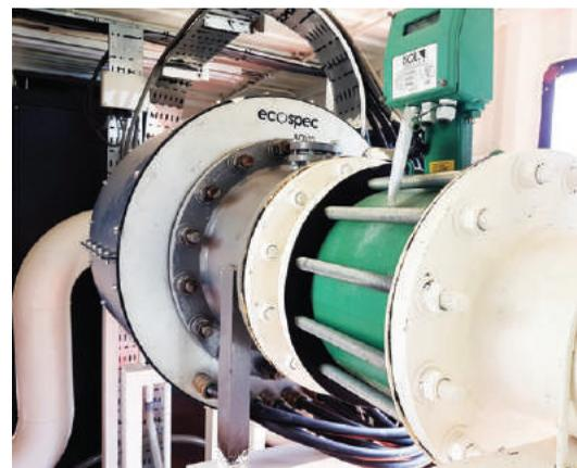
FIG. 2: Algae control unit (ACU) installed along the pipeline
