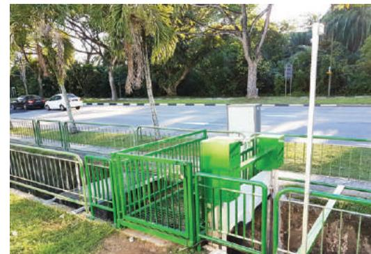
FIG. 2: The pollution detection and containment system installed at Upper Thomson Road
