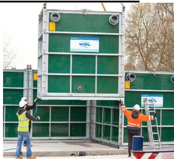
Installation of a modular WPL Hybrid-SAF
