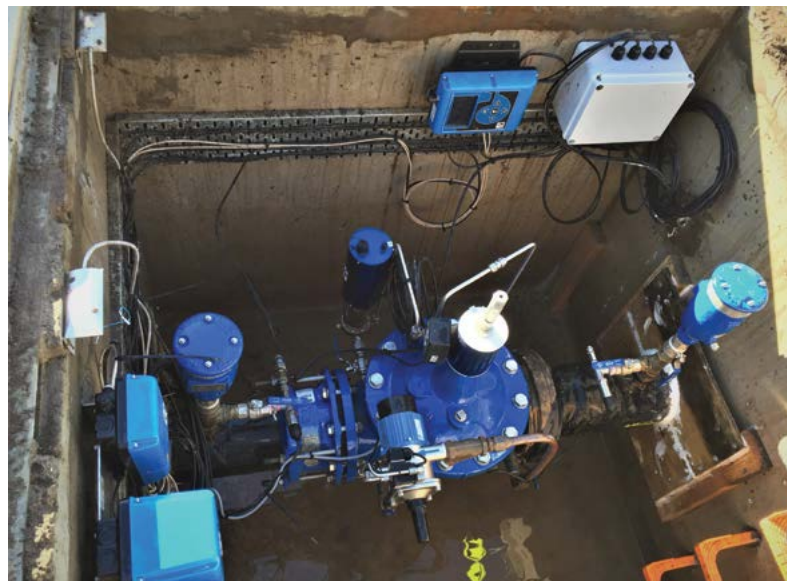
CWW installed several PRVs across the region
