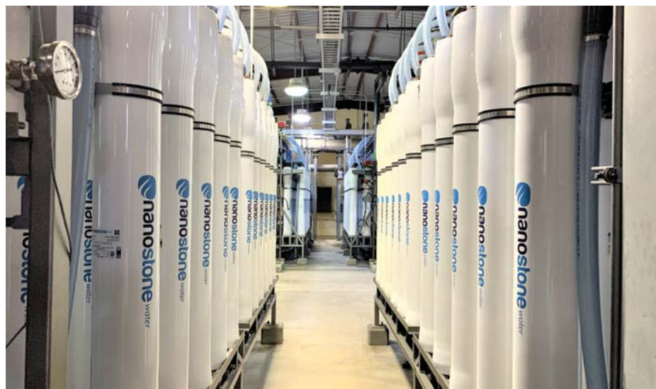
A TX drinking water plant installed with Nanostone ceramic membranes reached the daily capacity of 14.4 MGD
