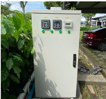
Figure 1. MES installed with IoT transmitter.
